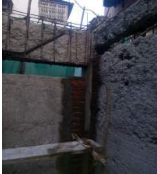
DAMAGED SLAB AND NEW SLAB CASTING DETAILS WITH BEAM / COLUMNS JACKETING IN IMAGES
