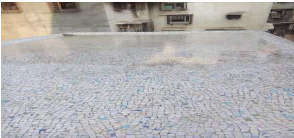
COMPLETED WITH CHIPS ON TERRACE
