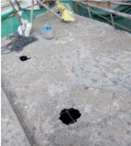
DAMAGED SLAB AND NEW SLAB CASTING DETAILS WITH BEAM / COLUMNS JACKETING IN IMAGES
